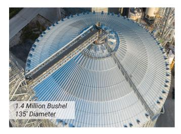
Sukup million bushel bins also feature a 16' or 21' flat deck around the peak of the bin. This provides more area to attach catwalks and conveyors as well as more room to work, making it safer to service.
