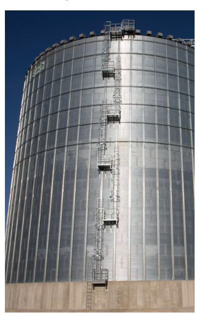
Sukup offers ladders and cages with 22' offset platforms or stairs to meet OSHA requirements. Sukup ladders feature continuous handrails and rungs that are securely fastened, so they can't turn.
